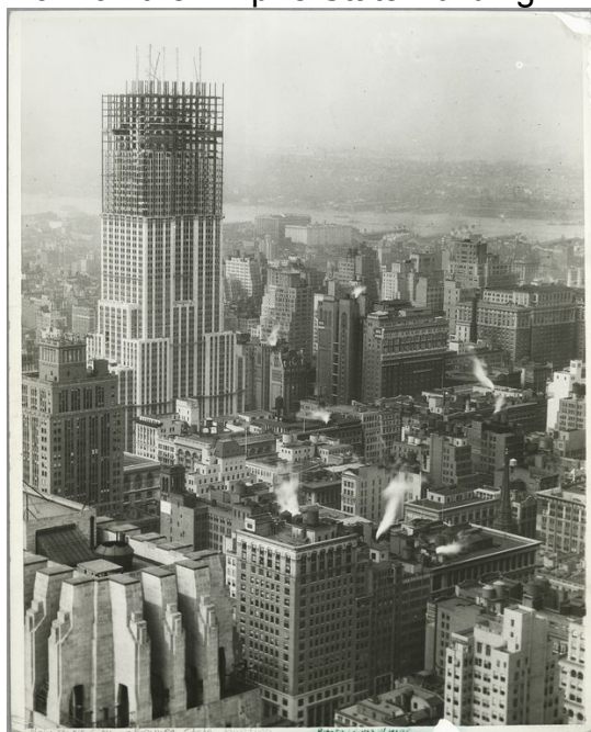
Empire State Building under construction 1931
